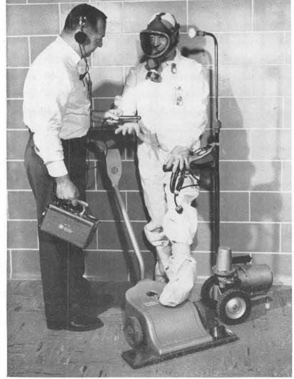
"TAKE ME TO YOUR METER," says Verne McNabney (right) as he and Bob Hanzel display radiation monitoring equipment used by the Health and Safety Section (8241-3) at Livermore Laboratory. New machine at right collects airborne radioactive and toxic particulates; machine under Verne's foot monitors alpha radiation on floor; and Bob holds conventional geiger counter. Verne wears protective equipment, including a respirator, in addition to a lapel air sampler, and a pocket dosimeter.
